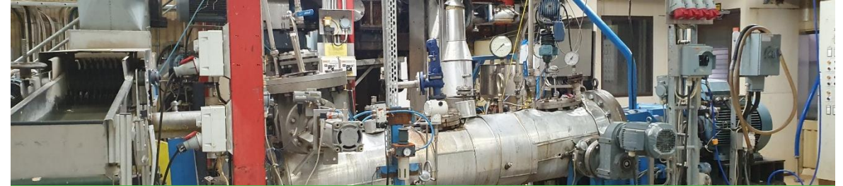
Fiber Technology Center, Sundsvall Sweden
